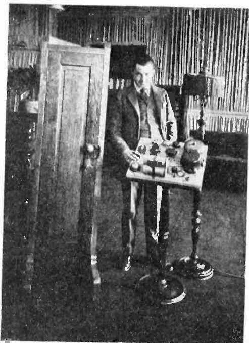
Edward H. Smith, director of WGY players, with the bell board and door used to produce sound atmosphere in radio drama. The exit and entrance of characters are indicated by the sound of the closing door. There are door bells, telephone, clock chimes, etc., on the board.
